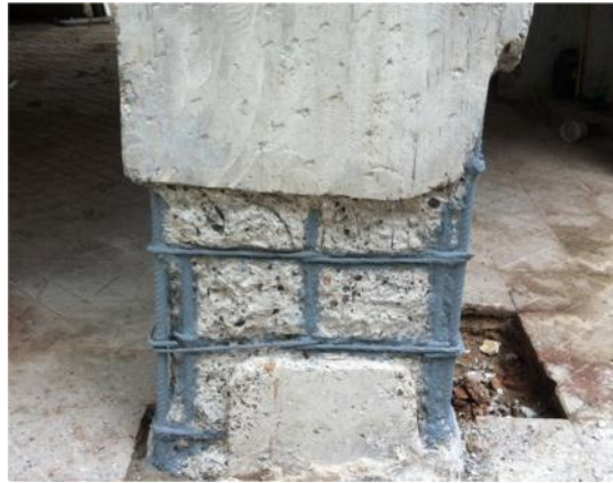
TYPICAL IMAGE OF SURFACE PREPARED RCC MEMBER
